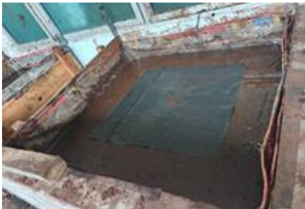
Figure 2: Research Location and Woven Geotextile Reinforcement
