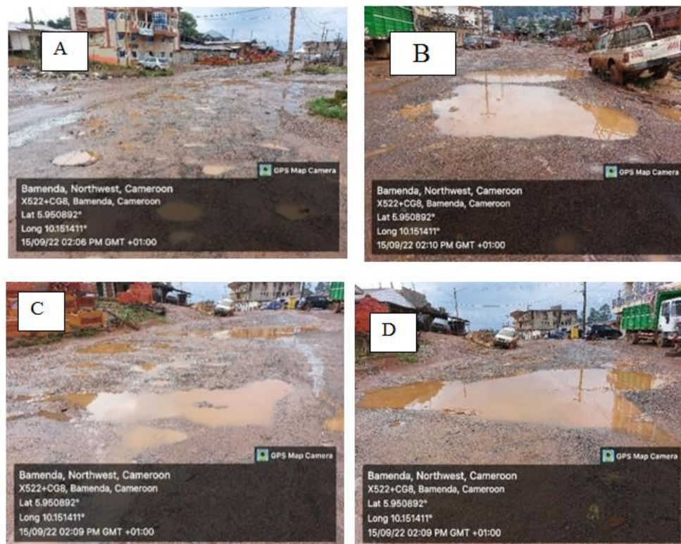
Fig. 9. State of streets characterized by potholes in Metta Quarters, Bamenda II Sub-division
