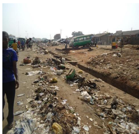
Figure 2.1. Refuse disposal along roadway
