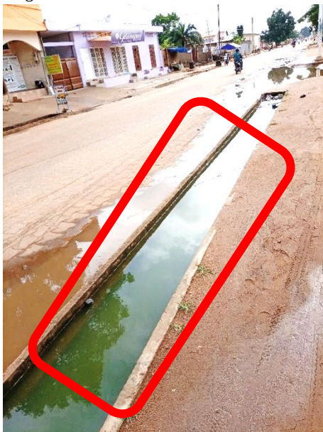
Figure2: Uncovered gutter
