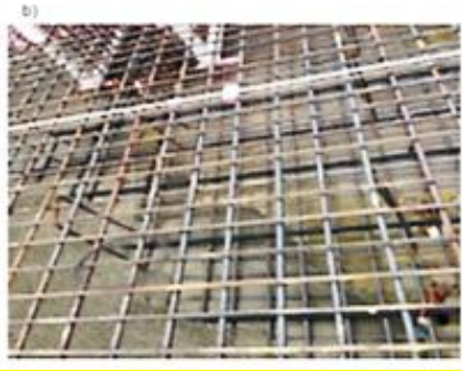
Fig. 6: Implementation of concrete loop a) placement of pipes b) covering pipes with concrete.
